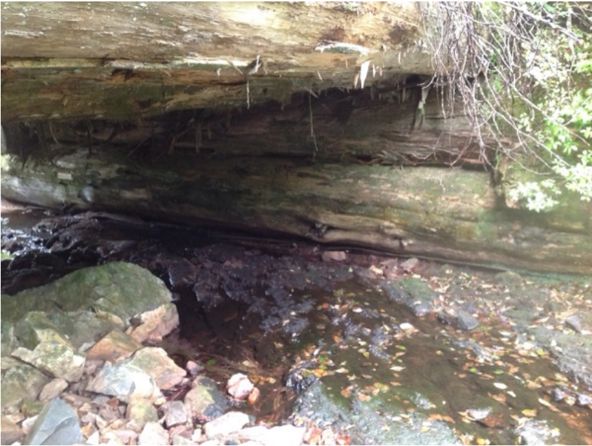
Right Bank Abutment when facing downstream
