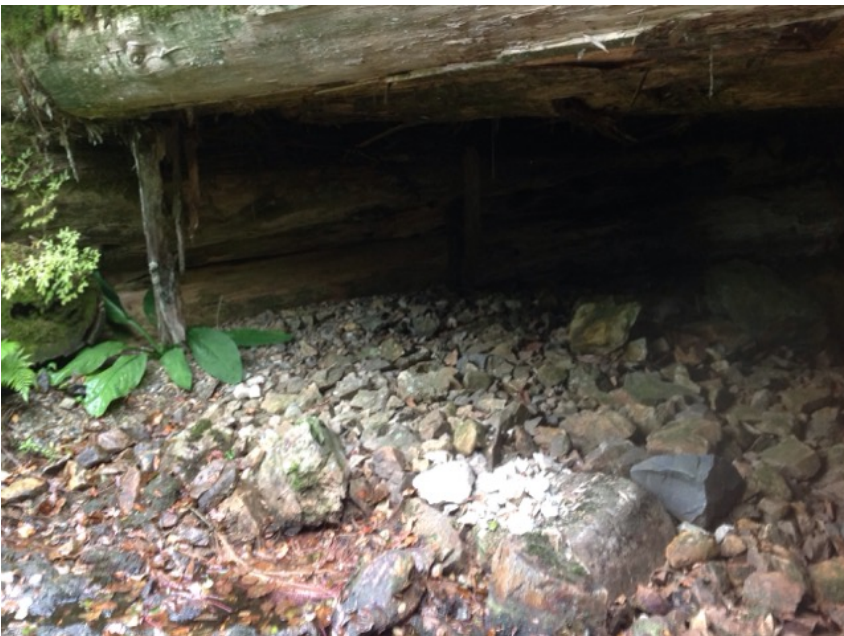
Left Bank Abutment when facing downstream
